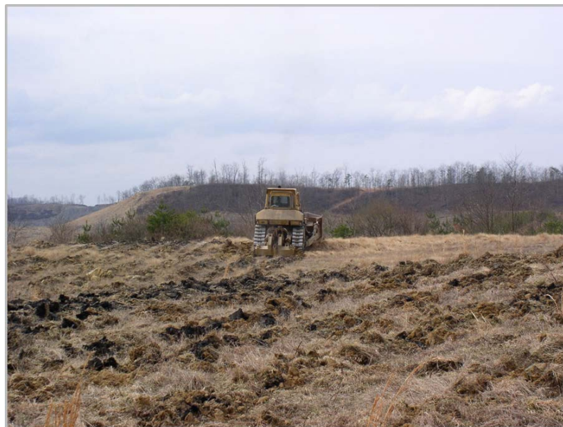
Figure 6. Ripping of compacted grassland mine soil.
