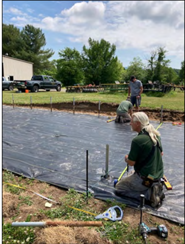
William Hamersky setting support tubes for the greenhouse at the new location at The DOF nursery
