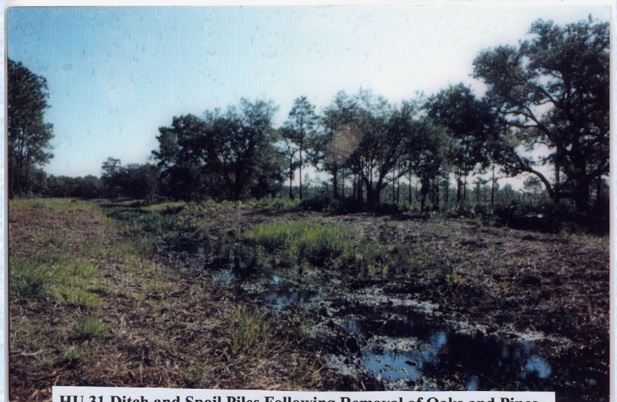
HU 31 Ditch and Spoil Piles Following Removal of Oaks and Pines, Prior to Filling of Ditch Sept. 1996
