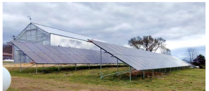
The new Meadowview greenhouse complete with solar panels.
